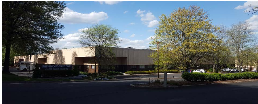
Rusten Corporate Park, Red Schoolhouse Road
